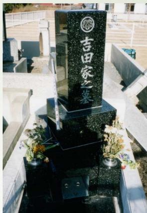
Figure 1 An example of rotation of a tombstone. A tombstone consisted of three rectangular granite blocks. Bottom one slid while the middle and top ones rotated together. During the 1994 Sanriku-Haruka-Oki, Japan, earthquake, 80 % of tombstones in a graveyard near the JMA Hachinohe observatory rotated in the same direction without overturning.
